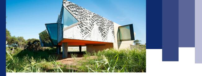
The building also includes all the sustainability features one would expect in a building of this nature, such as composting toilets, solar panels, natural ventilation, double glazing and full insulation. And, in another nod to its special purpose, construction took place over two bird migration seasons, with workers downing tools when some of the transient birdlife moved in for a lengthy stopover on the annual journey south to the Antarctic.
